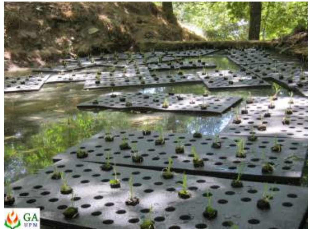
Green floating filters recently placed in Spain
